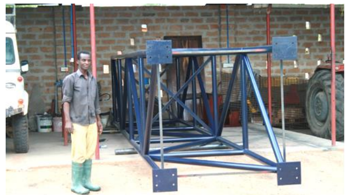
Water tower ready for setting into place
