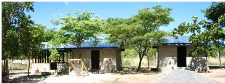
Toilet & laundry blocks
